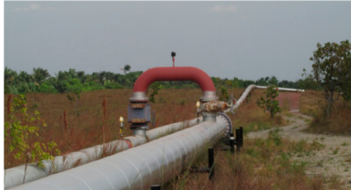
Figure 1. Loop in pipelines of heavy crude oil.
