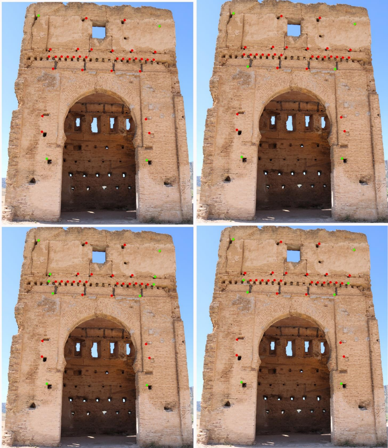
Figure 5. Configuration of the 4, 6, 8, and 10 control points (green points) from 34 collected points (red points). Clockwise from top-left
