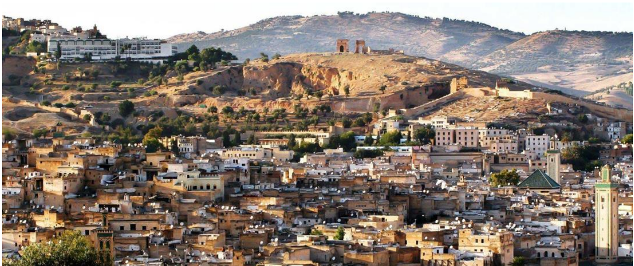
Figure 3. Location of the site at the top of the hill overlooking the old medina of Fès
