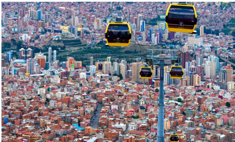
Figure 1: cable transportation system in Medellín, with circular section pylon
