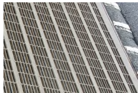
Photo 1: Grating on the bridge deck
