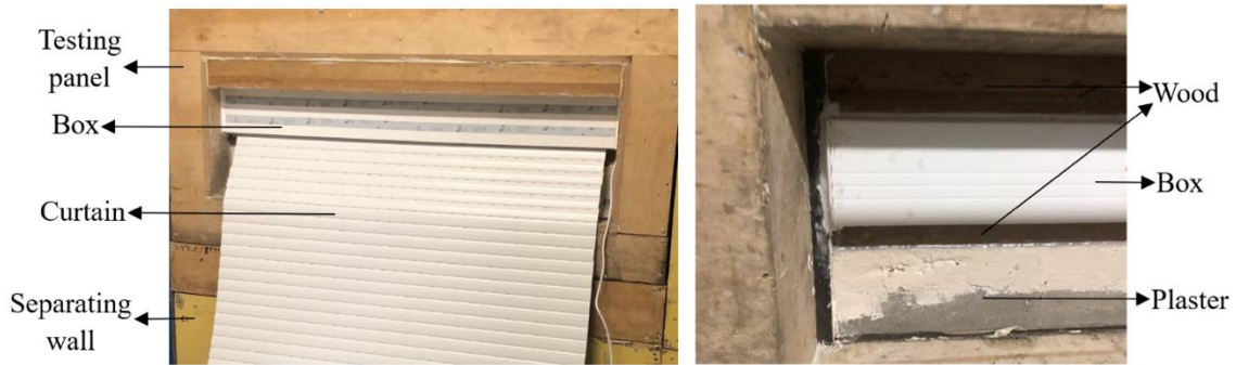
Fig. 6. Experimental test of the roller shutter box (a) front view (b) and rear view
